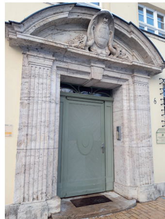
Portal, Travertin Ehringsdorf/Weimar
